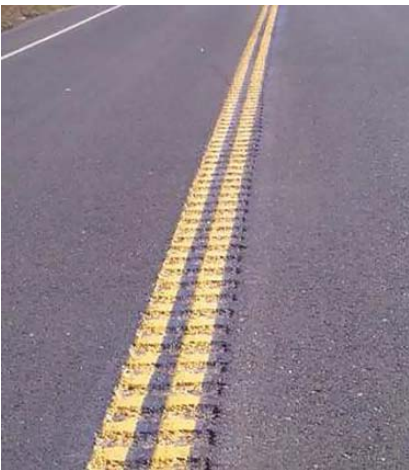
Centerline Rumble Strip
