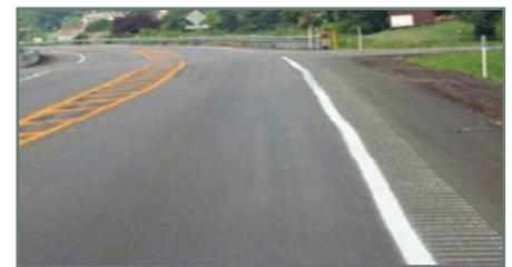
This photo shows the use of rumble strips on the outside shoulder and a painted median island.
