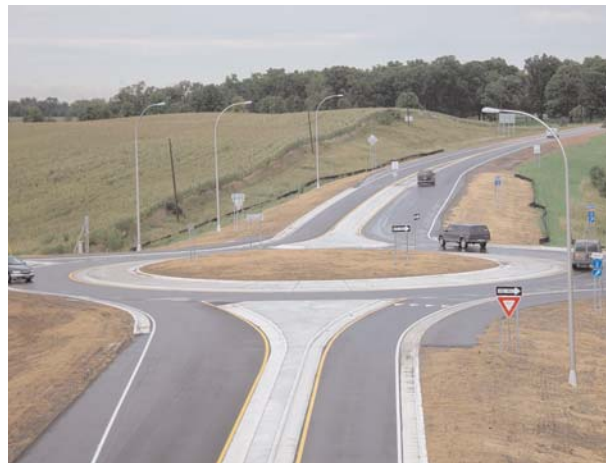
This high-speed roundabout at State Highway 13 and County Road 2 in Scott County, MN reduced the number of crashes to one. That crash involved a motorcycle that entered the roundabout at high speed and ran off the road.
