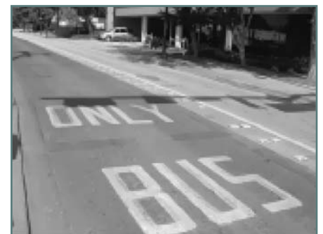
Bus Only pavement markings are used at an intersection in Orlando, Florida.
